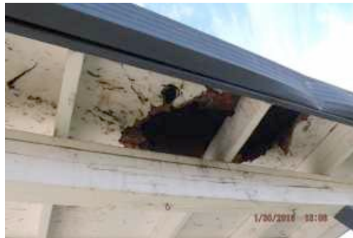
Boarded homes, holes in eaves, and bent gutters were just some of the deficits found at this Fairfield home.
